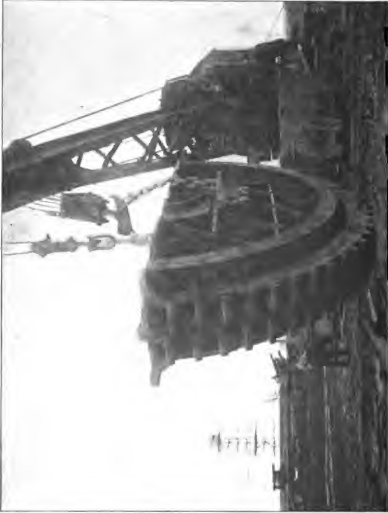
BASE RING OF THE 14-INCH, 45-CALIBER AMERICAN GUN MOUNT, MODEL "E" (SECOND STEP OF INSTALLATION).
